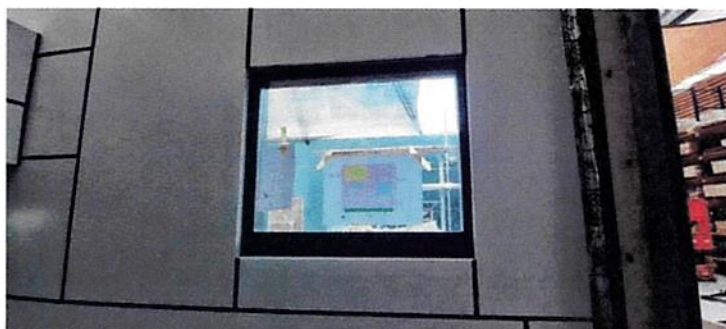
Figure 1: Photo of Panelab System with window and jointing
